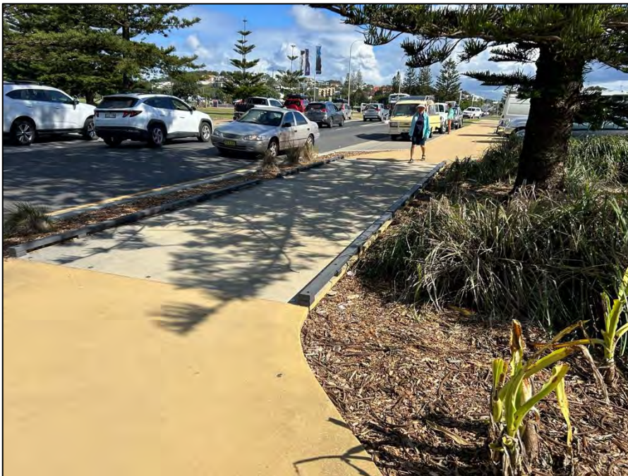
Figure 12 Example of a raised path with pier and beam design within the TPZ of a Norfolk Island Pine at Coffs Harbour Jetty.
