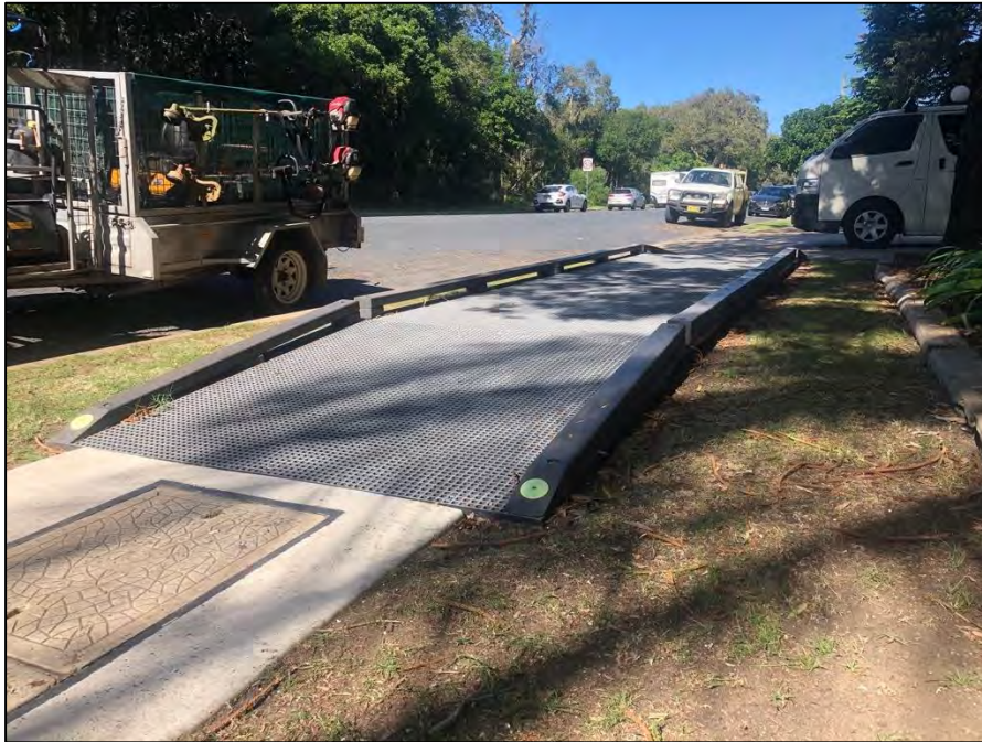
Figure 11 Example of a raised path with pier and beam design within the TPZ of a Norfolk Island Pine in Coffs Harbour.
